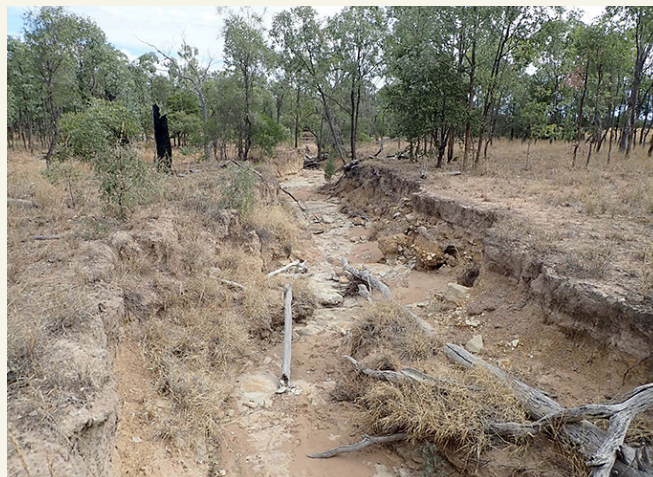
Image 2: This gully has eroded to the depth of underlying rock.
