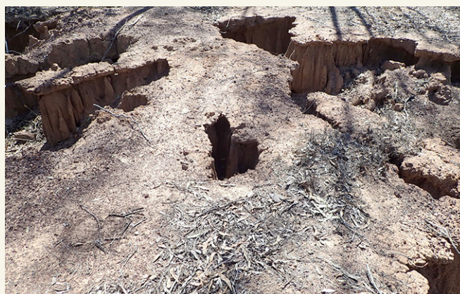
Image 4: Tunnelling is common in dispersive soils.
