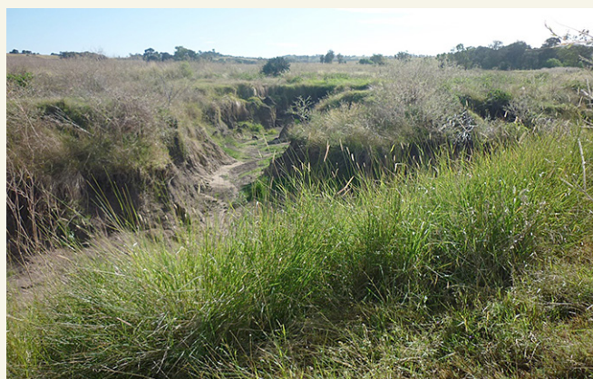
Image 1: Large gully up to 3 m deep before battering.
