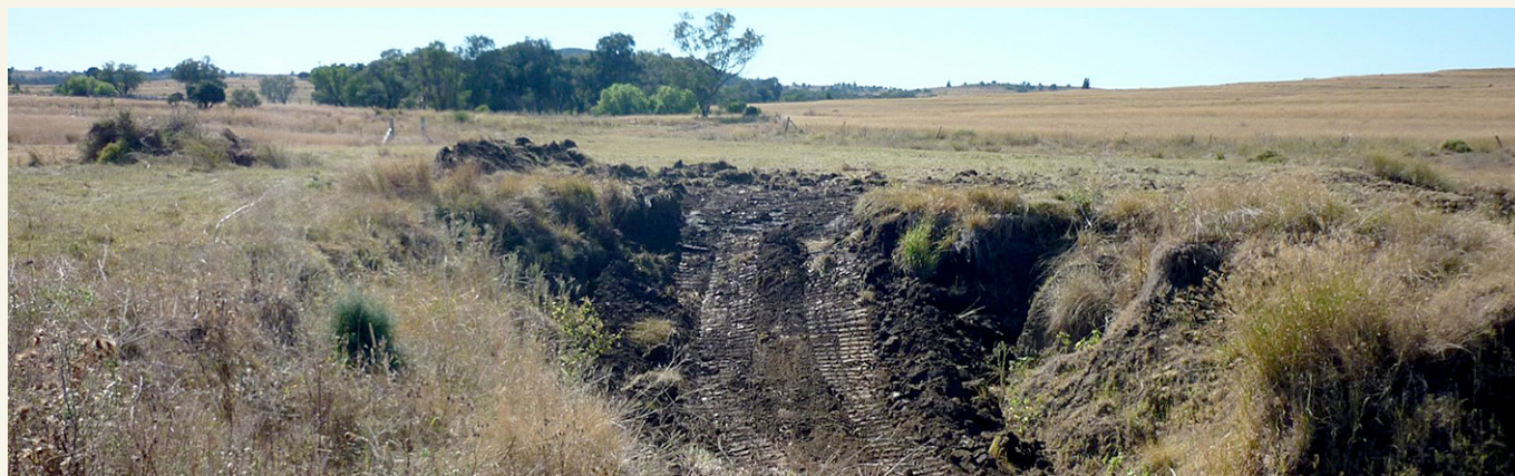
Image 3: Forming an earth ramp to batter the gully head.
