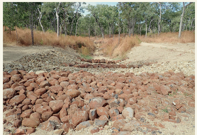
Image 2: Gully rehabilitation works in North Queensland.
