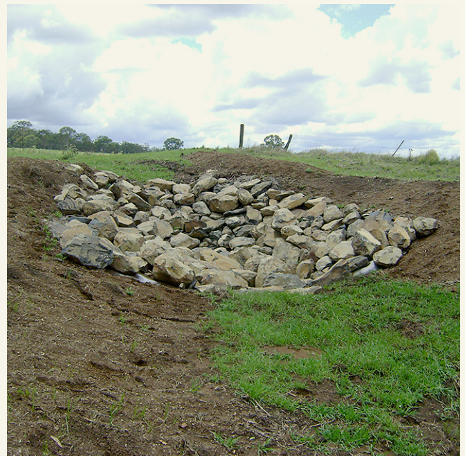
Image 4: Chute for controlling eroding gully head.
