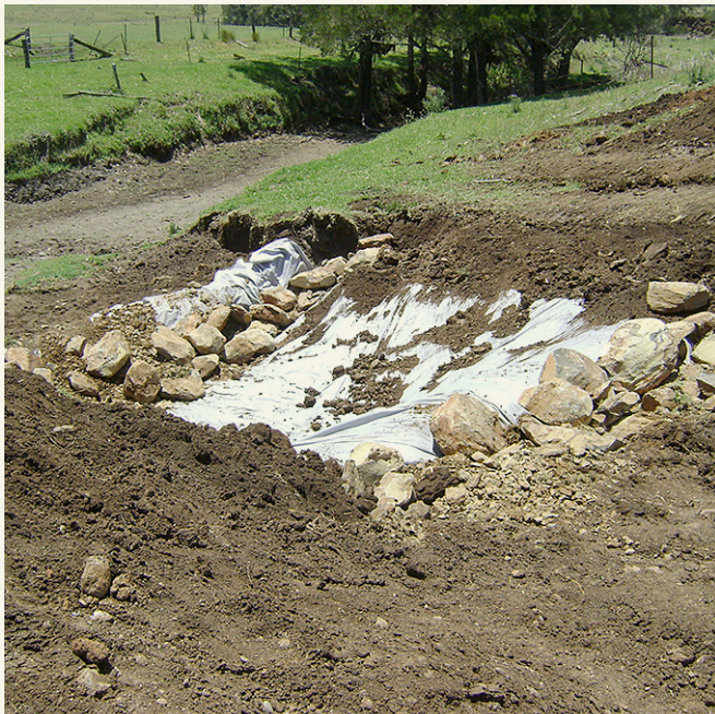
Image 3: Rock chute construction.
