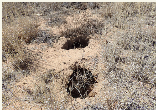
Image 5: Tunnel erosion in a sodic soil.
